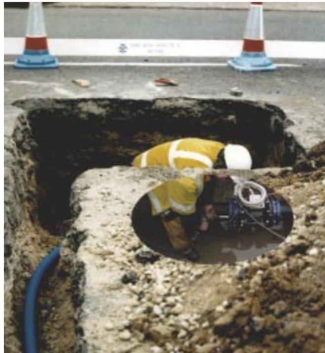
Underground Installation of AquaMaster™
