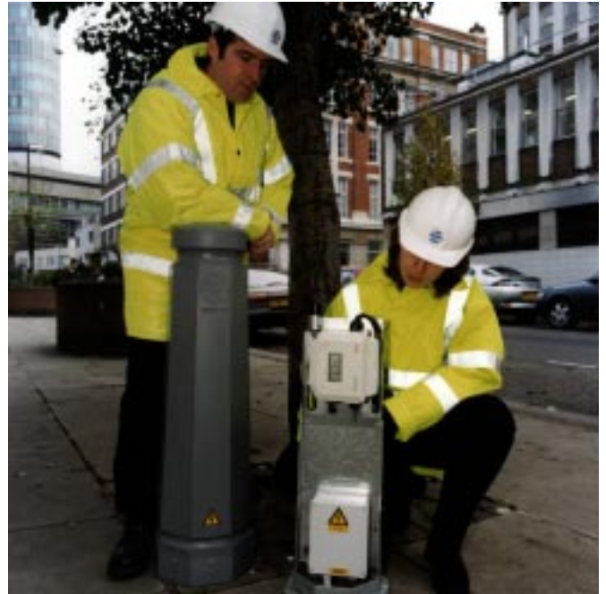
Typical District Metering AquaMaster™ Installation
